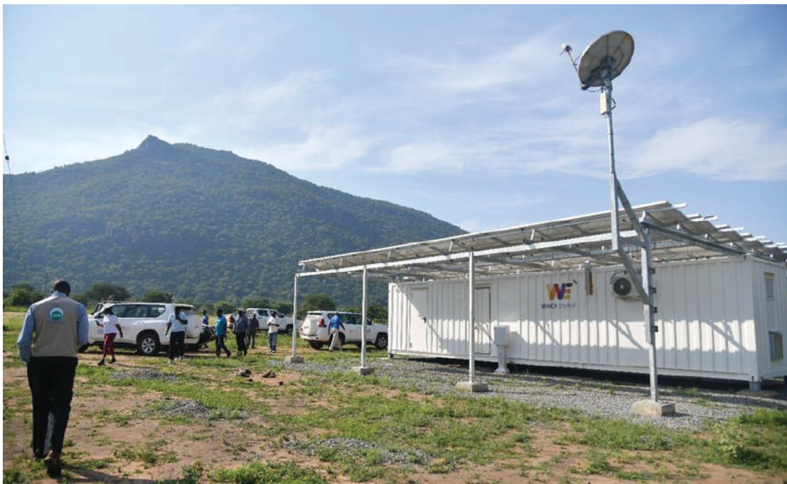
Figure 11 A 40kWp mini grid system in the Lamwo district, Northern Uganda. © GIZ
